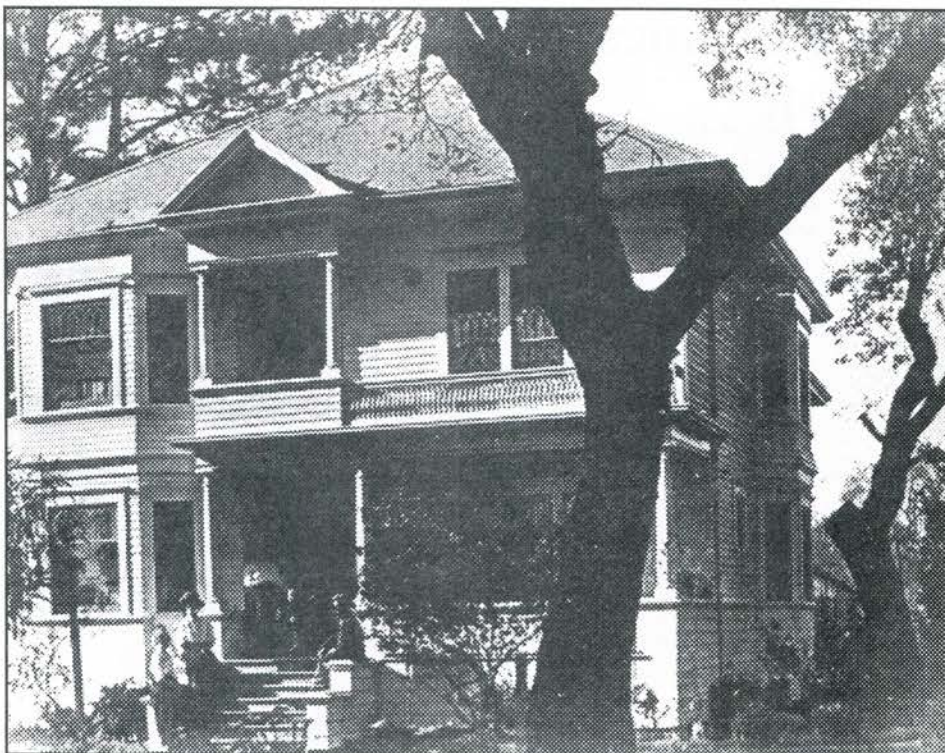
The Matheson House showing the 1904 remodeling
