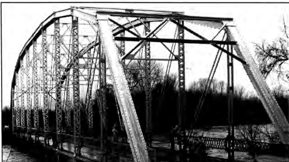
Lambert Bridge, 1952 flood. Photo provided courtesy of Howard and Adele Dicke
