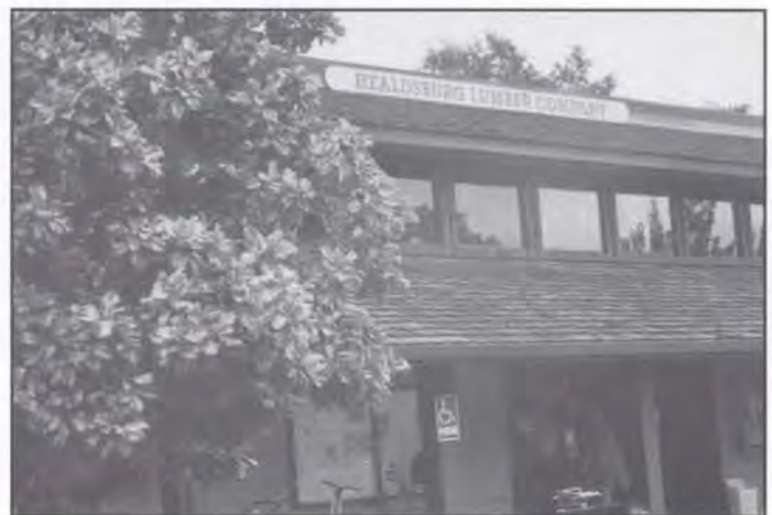
Present entrance to Healdsburg Lumber Company.
