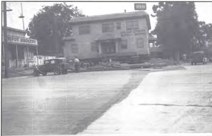
Buffi's Hotel moving from Healdsburg train depot to new location on West Street/Old Redwood Highway, 1937
