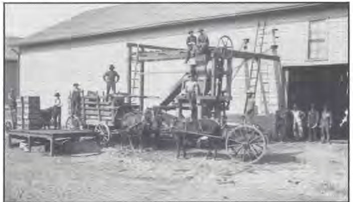
Geyserville Wine Association, Geyserville
