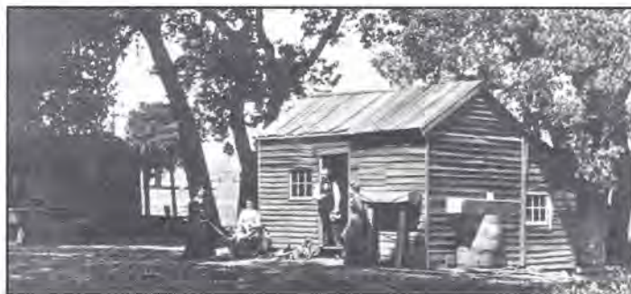
View of the first cabin dated 1851 at Dr. Elisha Ely's farm north of what became Geyserville taken on April 10, 1873, by Joseph H. Downing, photographer from Healdsburg. The cabin exemplifies the split-redwood log residence first constructed by pioneers in this area. Dr. Ely standing in doorway and Mrs. Ely in white seated to the left.
