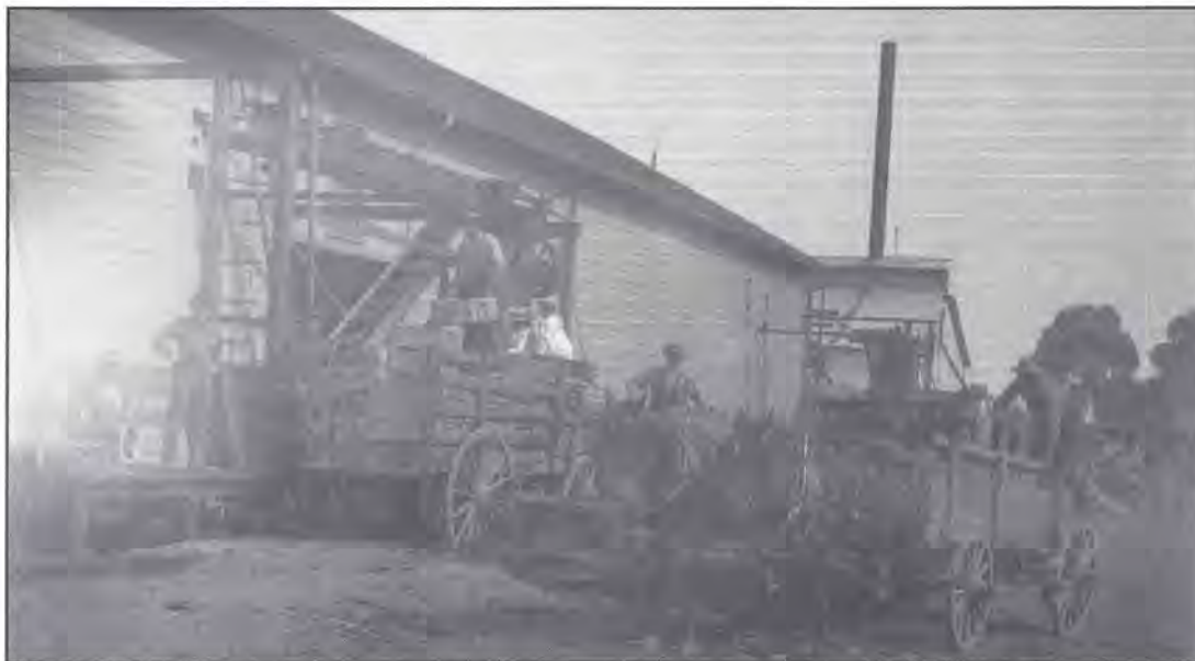
Geyserville Wine Association, Geyserville
