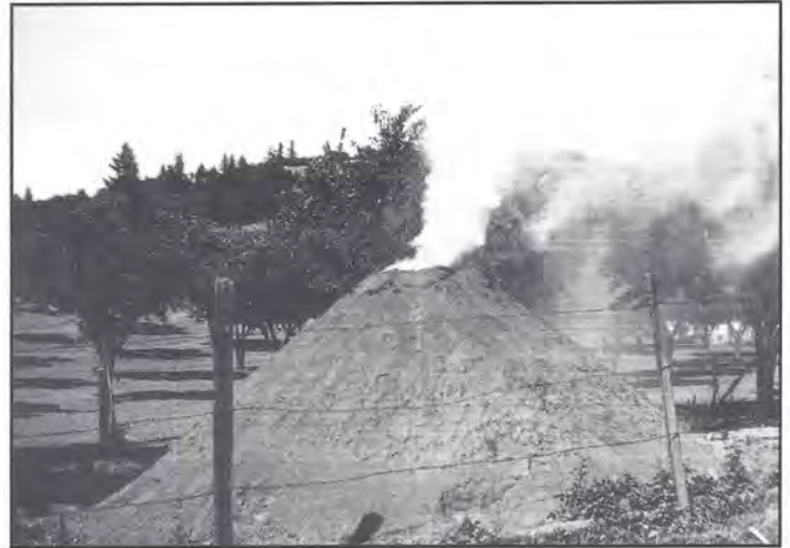
The smoke has stopped coming out the holes in the base of the mound. He is raking the dirt off of the mound of charcoal.
