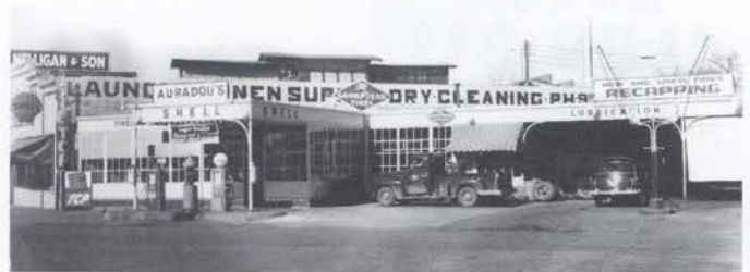
Auradou Shell Station, 1938
