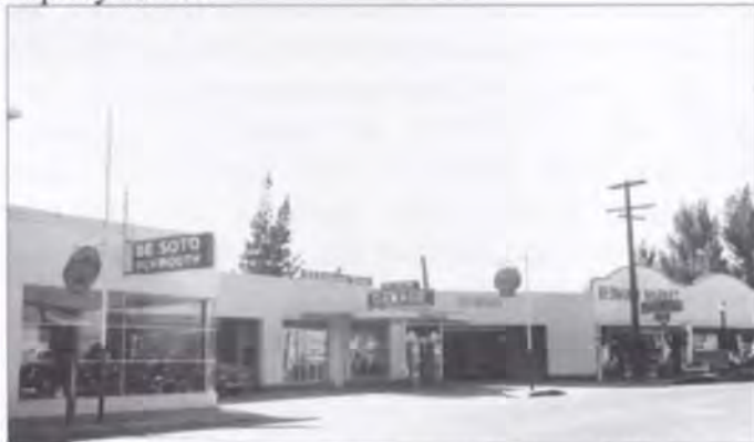
Remodeled garage buildings and Redwood Market
