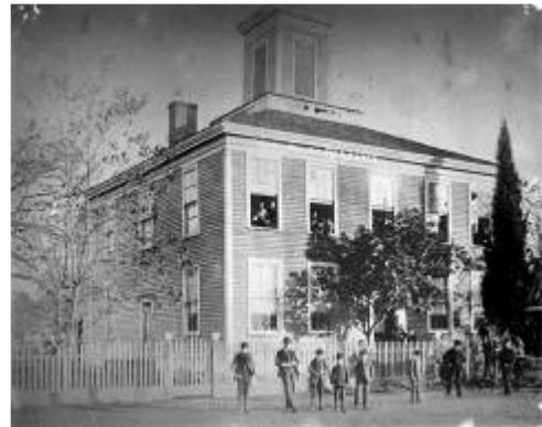
Healdsburg Academy, 1868, construction underway in 1857 (front page letter)
