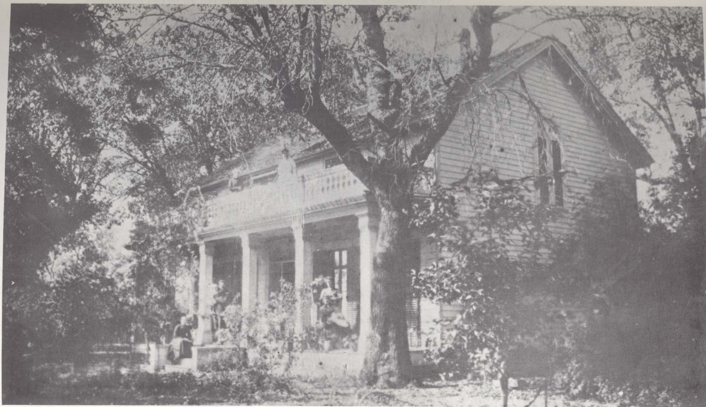
Home of Colonel Rod Matheson in Healdsburg, built in 1857 Once located on the site of the present Mrs. George Warfield home on Matheson Street
