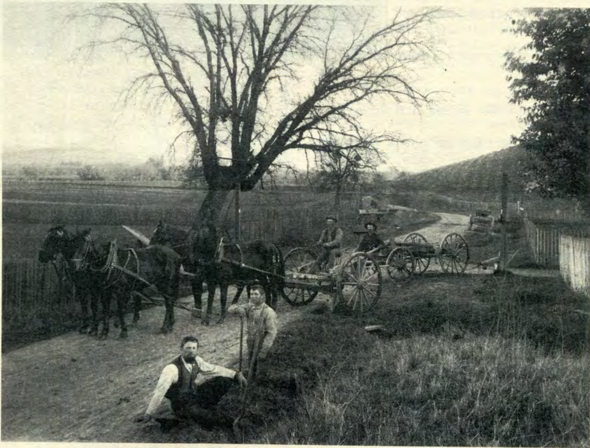
Road Scraper & work crew on Eastside Road circa 1890
