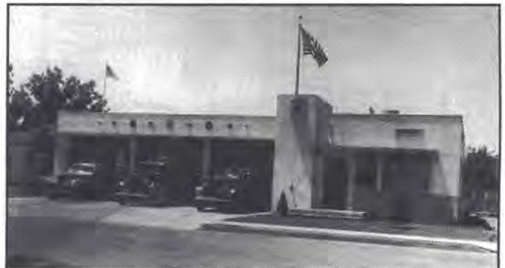
Healdsburg Firehouse on Center Street, July 4, 1942.
