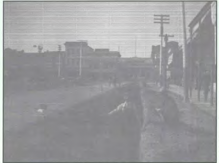
Digging a trench line for water lines, January 1900.
