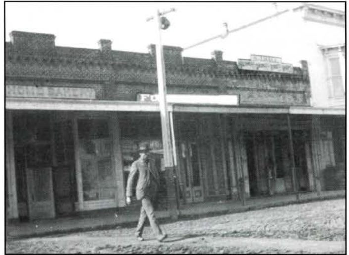
The Muller building, far right Hall's Saddlery next door on its left.
