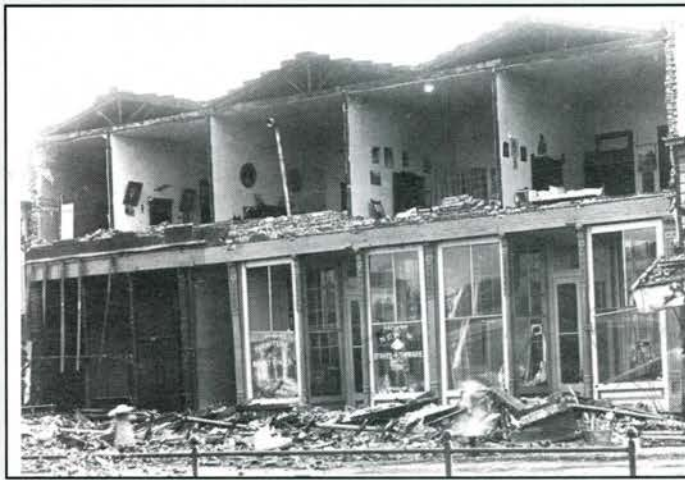
The Gobbi Building after the April 18, 1906 quake.
