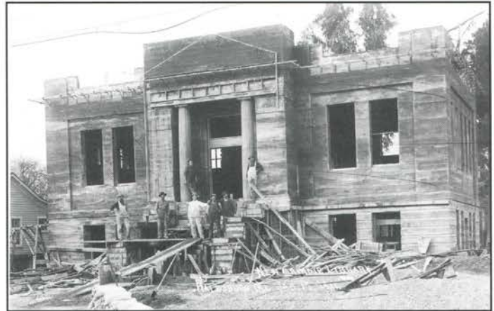
James Burgett (far right, in overalls) while constructing the Carnegie library Building in 1911
