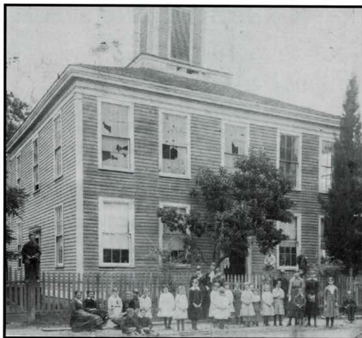
A schoolhouse in decline: The former Russian River Institute/Alexander Academy, 1870
