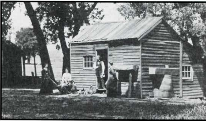
Elisha Ely's redwood cabin near Geyserville, built in 1851, exemplifies the type of split-log pioneer residence first constructed in this area. Joseph Downing photograph, 1872
