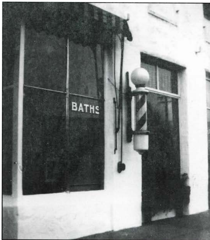
The barber pole outside the Sotoyome Hotel just prior to the building's demolition.
