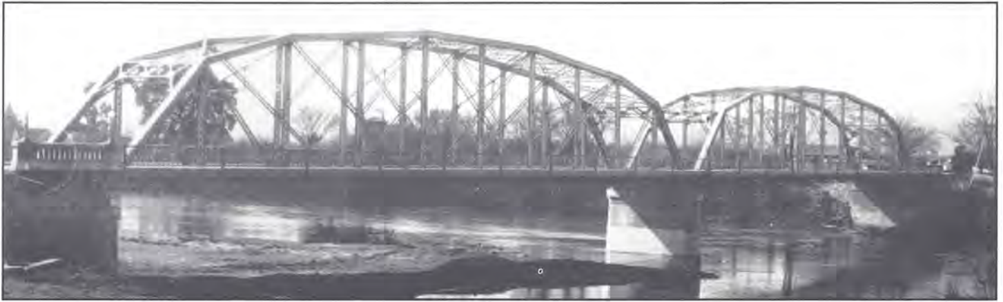
1921 Bridge, newly constructed.
