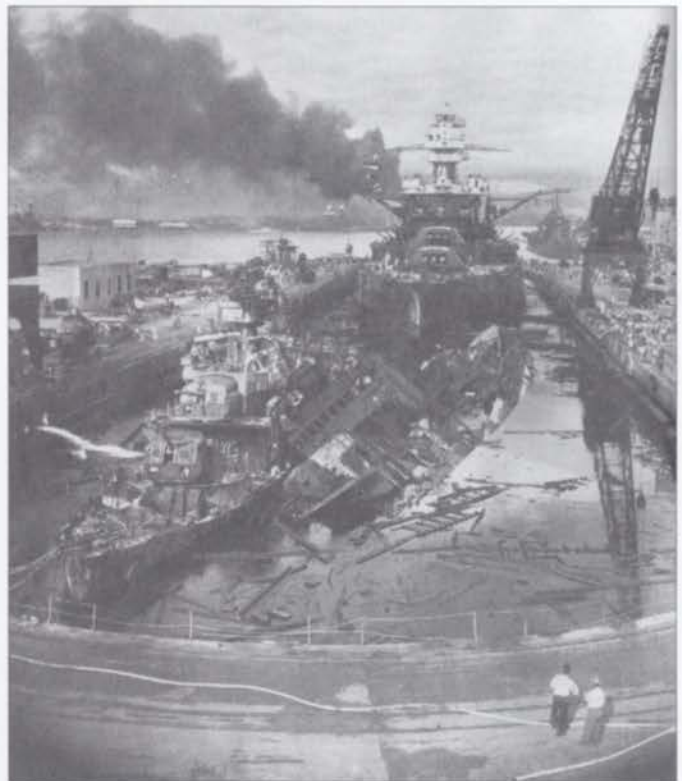
The U.S.S. Pennsylvania lies in a drydock behind the wreckage of the destroyer Cassin (right) and Downes (left). Flagship of the U.S. Fleet, the Pennsylvania suffered relatively light damage and was repaired soon after Dec. 7. The Cassin and Downes were both lost, but their machinery and equipment were transferred to new hulls. U.S. Navy photo, National Archives Collection, December 7, 1941.
