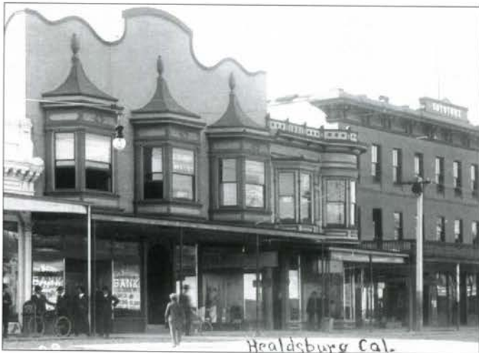
West Street (Healdsburg Avenue), northwest of Plaza, 1904 and 1906
